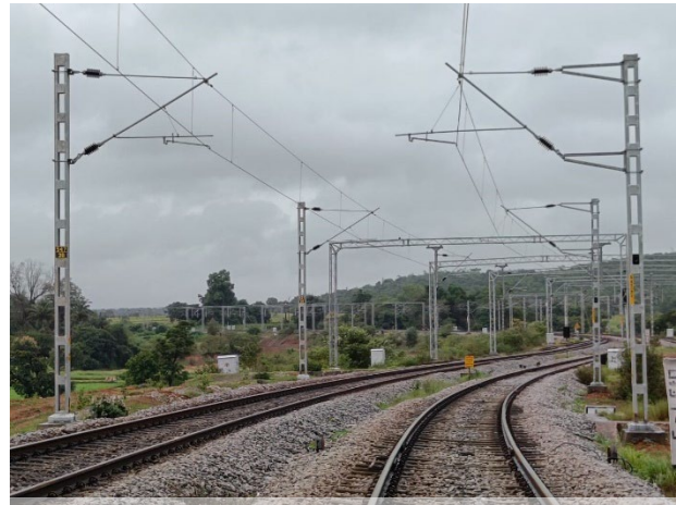
Hubli - Tinaighat Railway Electrification project, Karnataka
