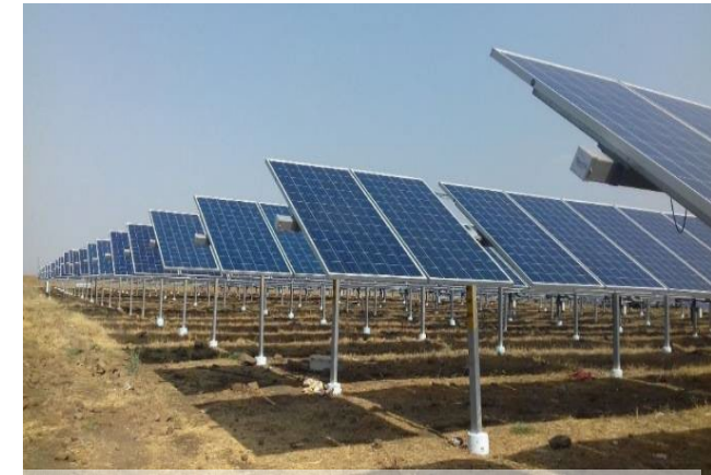
30 MW Tracker Based Installation, Andhra Pradesh
