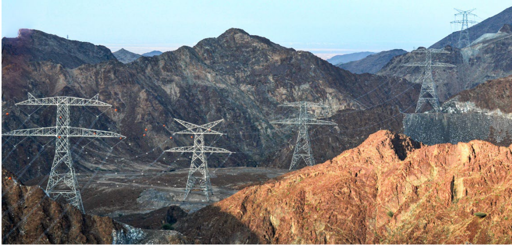
400 kV IBRI-New Rustaq O/H Transmission Line, Oman
