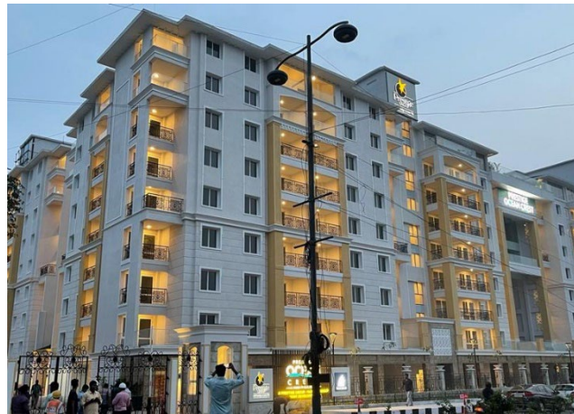
Construction of luxury residential project in Goa
